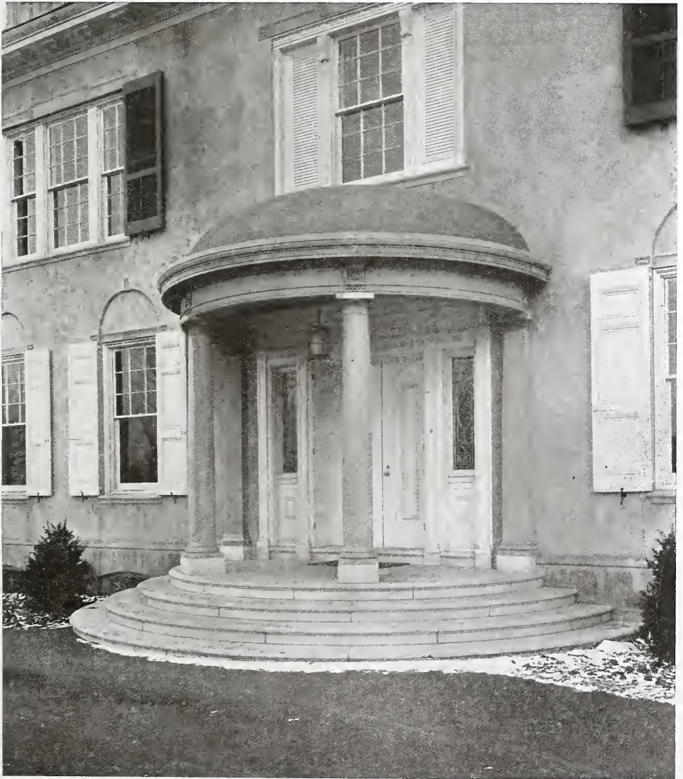
ENTRANCE DETAIL—THE COLTON RESIDENCE. Bryn Mawr, Pa. Horace Wells Sellers, Architect.
